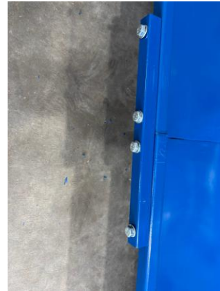
Support fasteners installed through the trough
