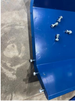
Install all flange fasteners at each trough joint
